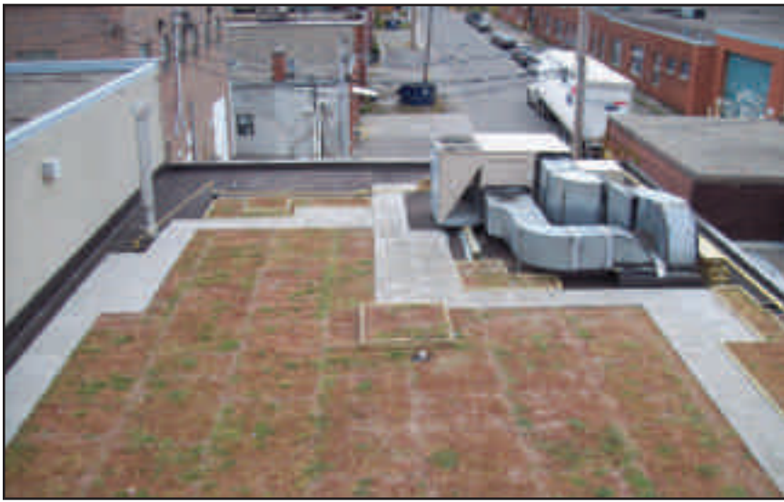
The finished green roof on the Drum Artz Centre.
