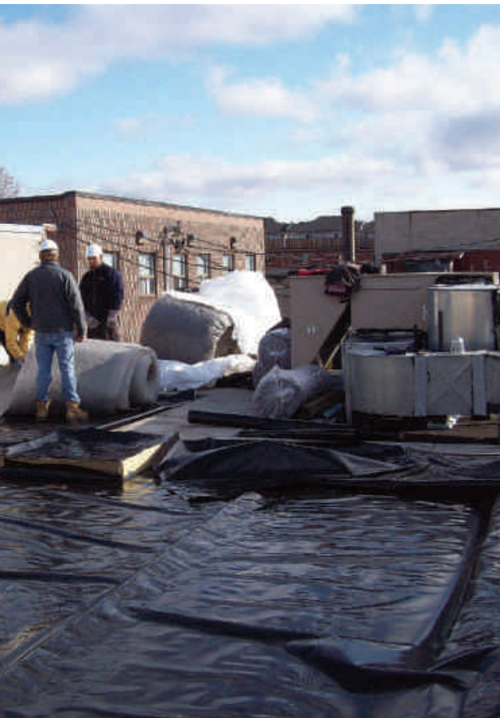
Laying the membrane, a 2-ply modified bitumen.
